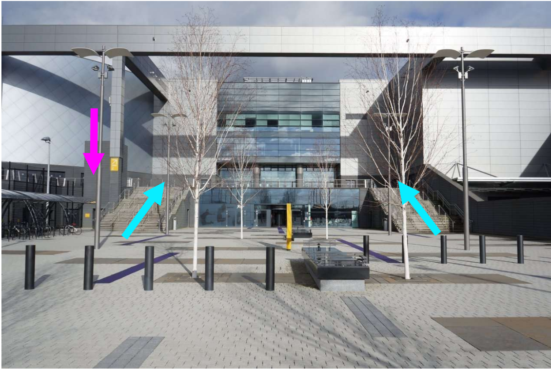
Emirates Arena, Main Entrance
